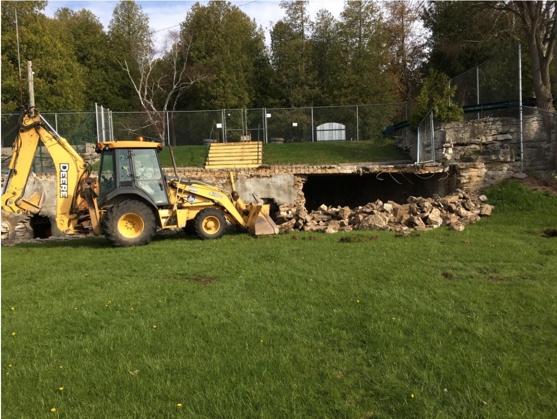
Demolition of Bear Pen at Bruemmer Park Zoo
