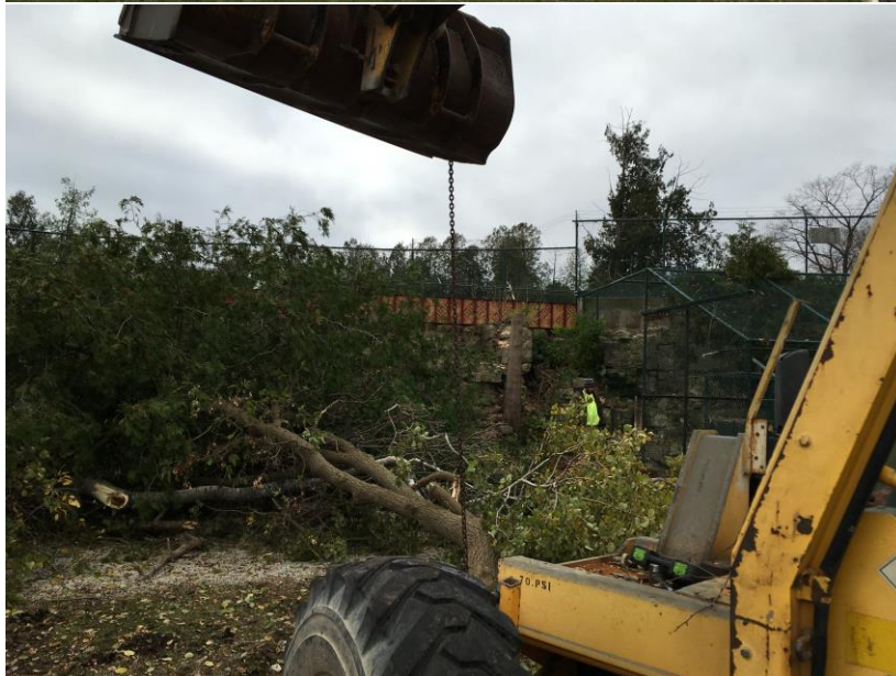
(Bobcat Exhibit Construction at Bruemmer Park Zoo)
